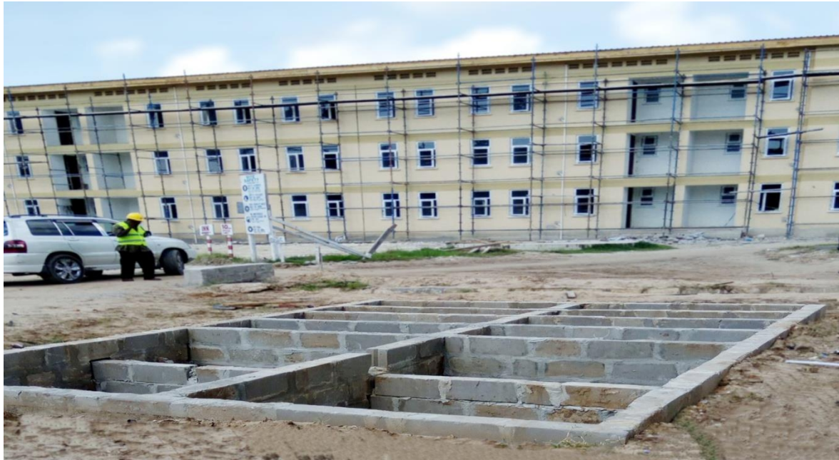
Photo 1. 1 Construction of Anaerobic Baffle Reactor at Kunduchi Senior police Houses
